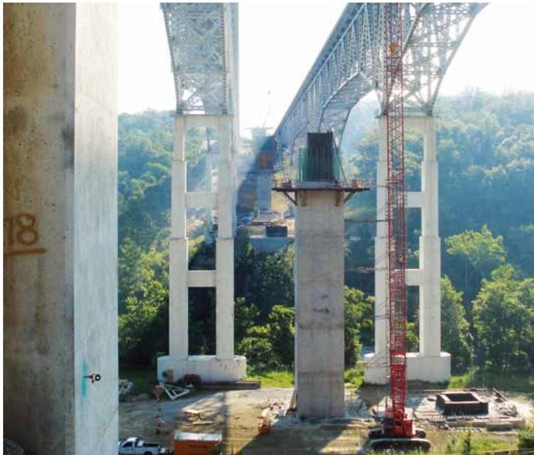
*Each of the twin structures consists of a single cell, variable depth box girder. Photo courtesy of James E. Barnhart, Ohio Ready Mixed Concrete Association.*
