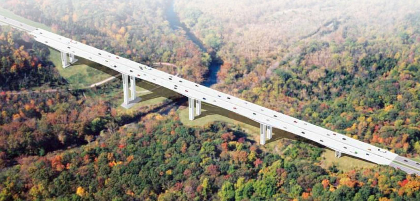
*Rendering illustrates the new bridge that consists of twin, six-span, cast-in-place concrete, variable depth, segmental box girders. Bridge rendering courtesy of HNTB.*
