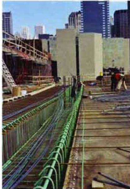
*Parking garage, balconies and terraces, all areas exposed to weather and de-icing salts, were specified with epoxy-coated reinforcement to extend service life.*
