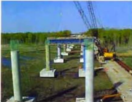
*A cap covers the columns and joins them together. Girders are placed on the capped columns. Pre-cast panels and cast-in-place concrete are used for the bridge deck. Approaches use pre-stressed concrete girders and the main span of the bridge is post-tensioned.*
