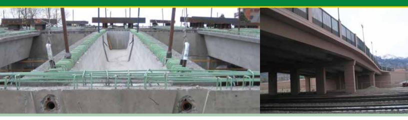
Colorado Springs needed a new bridge to relieve congestion and provide added access to the downtown area as well as project a new welcoming image for the city. These goals were reached with a design that featured a spliced, post-tensioned, precast concrete superstructure with an innovative prestressing layouts and variable cross-sections to accommodate a unique erection methodology. The project was completed in only 10 months.
