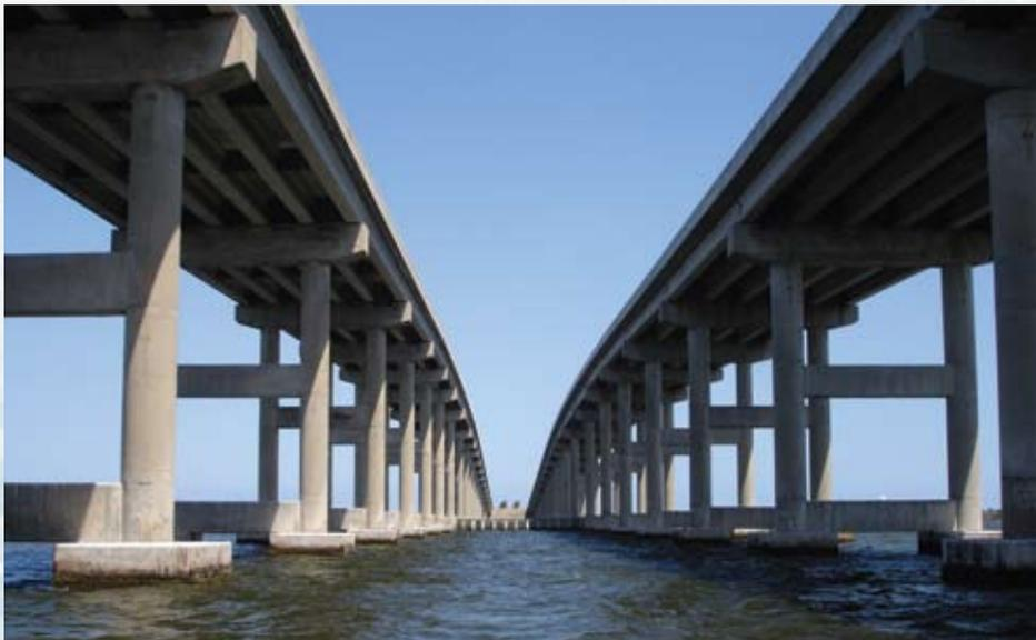
Figure 4: Companion bridges containing either black (left) or epoxy-coated bars (right) in Melbourne Florida.
