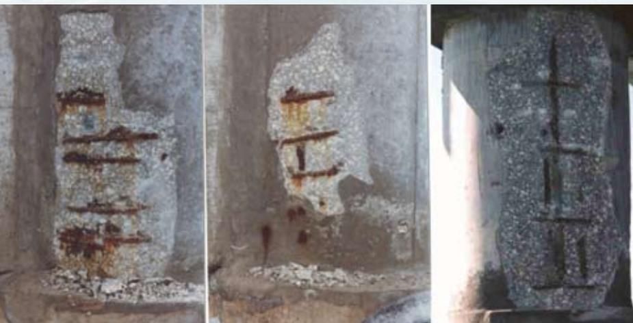
Figure 1: Typical spalls observed in bridge piers<sup>(1)</sup>.
