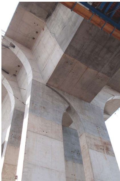
Main river piers are 3 ft by 9 ft 6 in. and extend 45 ft above the top of the ice breaker to the pier table. Photo: FIGG.
