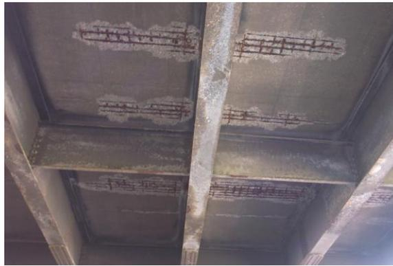
Figure 6: Deterioration of bridge deck using uncoated bars as bottom mat and epoxy-coated bars as the top mat
