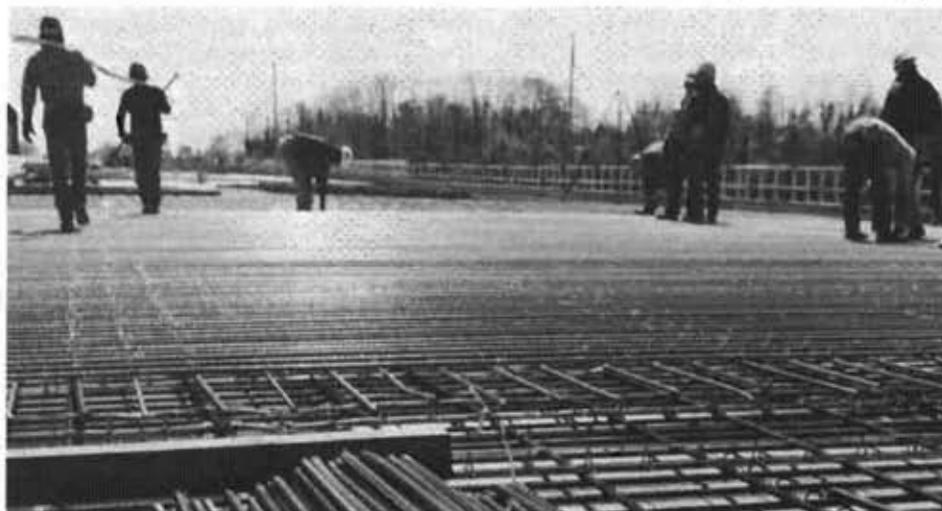
Earlier this year, the FHWA in docket 83-1, proposed revisions to 23 CFR.650 relating to concrete bridge decks. This, in effect, made the coating of reinforcing steel by epoxy or metallic means an option of each state.
