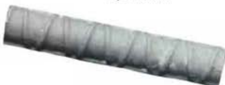
Actual sample of original 8 year old epoxy-coated rebar. Absolutely no sign of corrosion.
