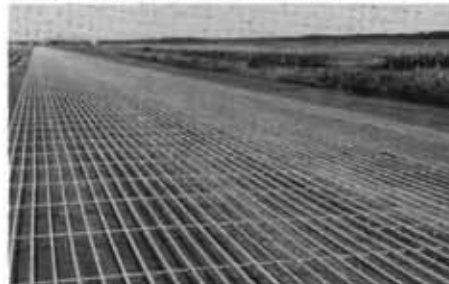
Epoxy-coated rebar was set on bar chairs for close placement control.
