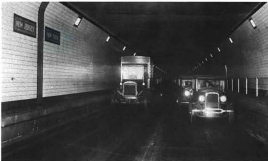
Deicing salts are not the only cause of corrosion! Imagine cars and trucks, as in this 1929 scene, spewing corrosive exhaust every day for 60 years. No wonder the unprotected ceiling gradually began to deteriorate.
