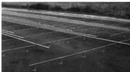
Longitudinal epoxy-coated rebar were set on transverse epoxy-coated rebar with prefabricated epoxy-coated chairs.
