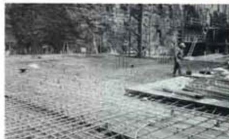
Close-up of the placement of the epoxy-coated rebar on the parking ramp far below street level.
