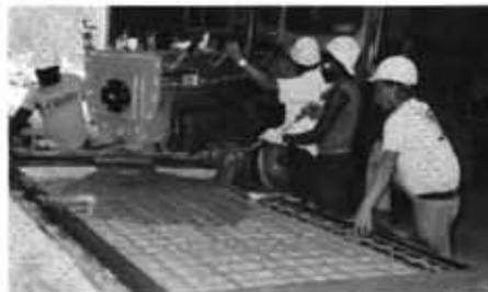
Concrete is poured over panels reinforced with epoxy-coated rebar.
