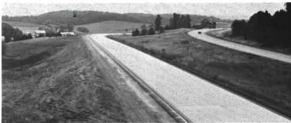
Completed section of smooth, continuously reinforced concrete pavement.
