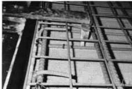
After the slurry has set, the reinforcing steel is positioned on top and the 4-3/4 inch layer of concrete is poured.
