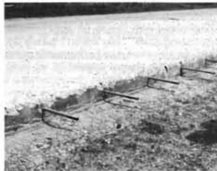
The old pavement was widened at the same time as overlay was put down. To tie the widened section into the old pavement, epoxy-coated rebars were inserted in drilled holes as show.
