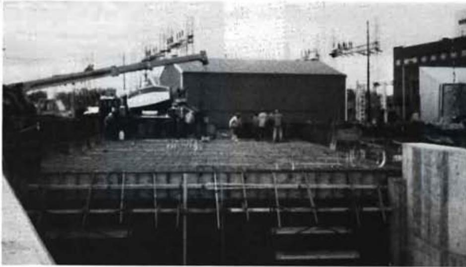
Pouring the deck over the water treatment plant. All rebar is epoxy-coated.
