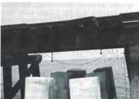
The six pile concrete bent and steel bent in place ready to receive poured-in-place concrete cap.
