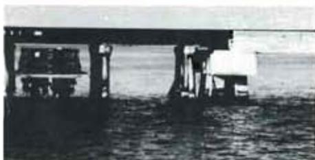
Closeup showing new concrete section adjoining old, original wood span.
