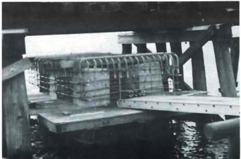
Rebar cage of Grade 60 epoxy-coated steel in place ready for forming and pouring.
