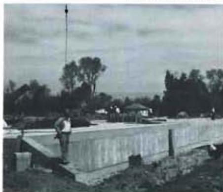
Flume was built on grade to facilitate construction and excavated for I-70 to pass beneath it.
