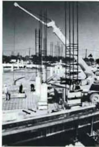
Level two of the garage with epoxy-coated rebar being placed.
