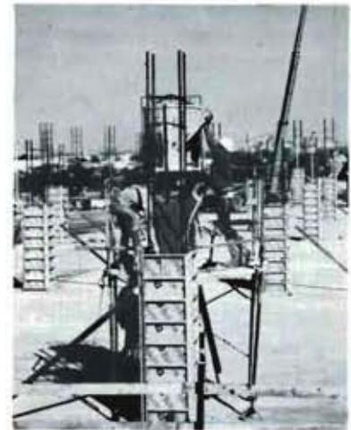
Forming the concrete columns for the 5-level structure.
