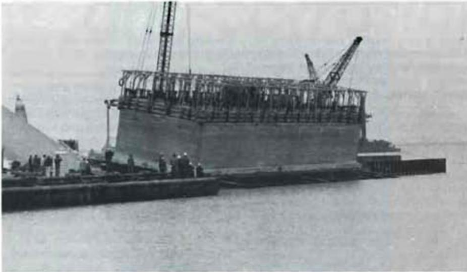
Launching completed 900-ton concrete wharf.
