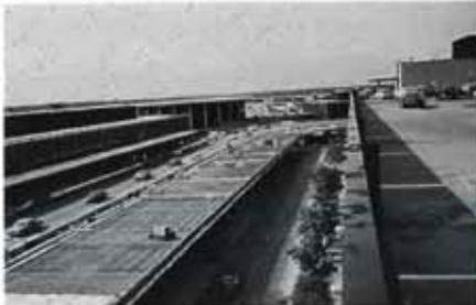
Passing Terminal 3, installation of the epoxy-coated rebar is nearly complete; ready for deck construction.
