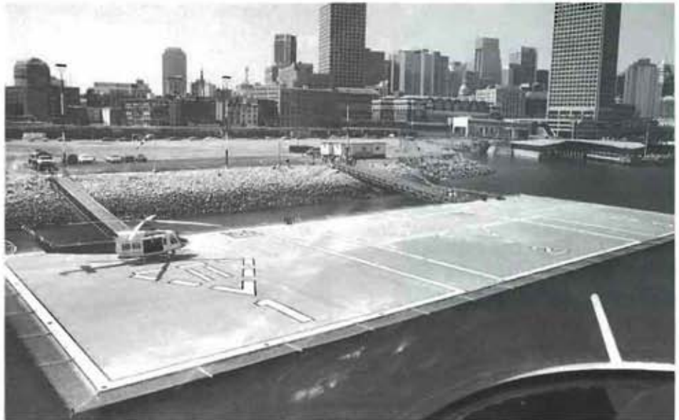
View of completed heliport from an incoming helicopter. Moored near downtown Vancouver, the heliport can be moved to another location if site priorities change.
