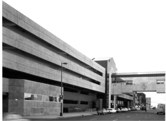
The City Center Parking Facility in Columbus, Ohio is a 1.4 million square foot structure built with a cast-in-place concrete frame and conventionally reinforced columns.
