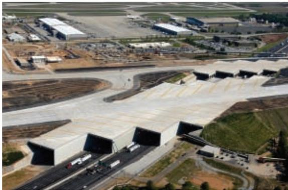
runway bridge measures 1,200 feet long by 486 feet wide, and its taxiway bridge is 450 feet long by 450 feet wide. While most aircraft touch down before they cross the bridged section, the bridge is designed to withstand an aircraft load well over the weight of a 1.04 million-pound wide-
