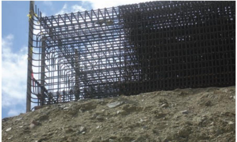
Reinforcing cage for Galena Creek Bridge Arch
