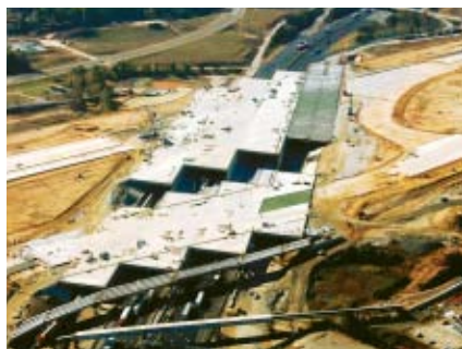
Aerial view of box culverts under construction
