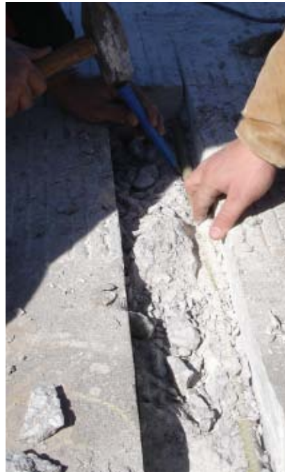
Extraction procedure of 15 year old epoxy-coated rebar used in this study
