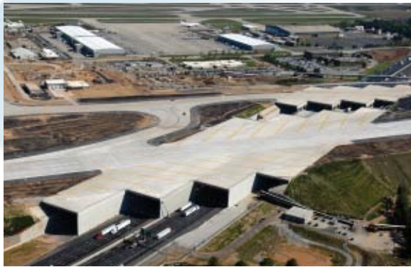
Aerial view of Interstate 285 and box culverts
