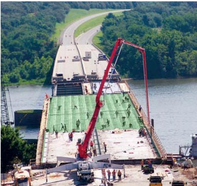
Epoxy-coated reinforcement before the deck pour.
