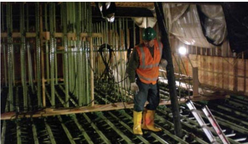
Epoxy-coated reinforcing steel bars inside a footing at the beginning of the concrete pour
