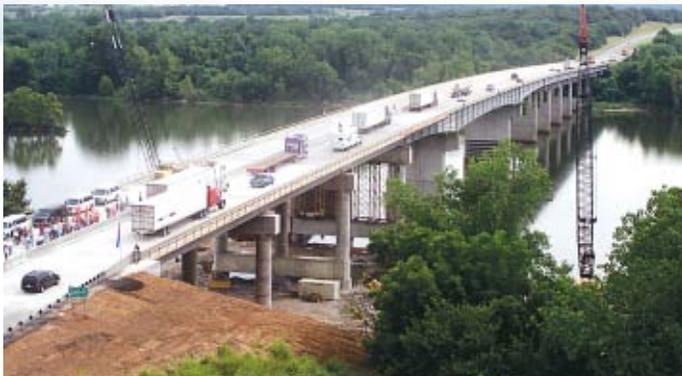
Recently reconstructed I-40 bridge in Oklahoma. Completed in 65 days using 235 tons of epoxy-coated rebar in both decks following a barge collision that collapsed the original bridge.
